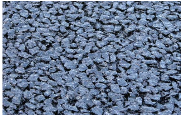
Figure 2.2 – Pavement surface immediately following paving and compaction.
