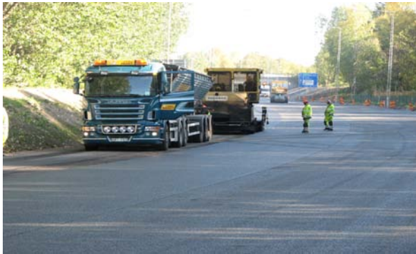
Figure 2.1 - Paving of asphalt-rubber OGFC in Norrköping, Sweden.
