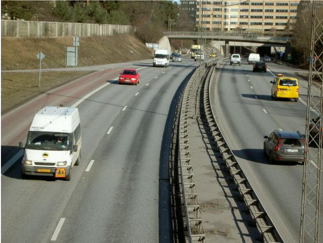
Figure 3: The fast lanes after one winter (GAP 16 to the left, ABS16 Nypol 50/100-75 to the right)
